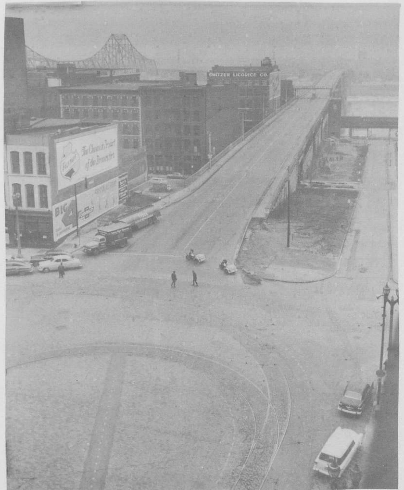
Washington Avenue looking east from Fourth Street showing traffic on Eads Bridge being cleared during Red Warning. (Photography by Linck, St. Louis Post-Dispatch.)
